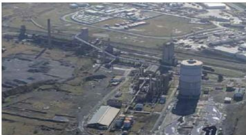
South Bank coke ovens
