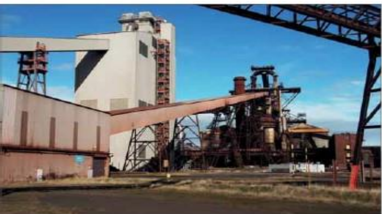
Pulverised coal injection plant
