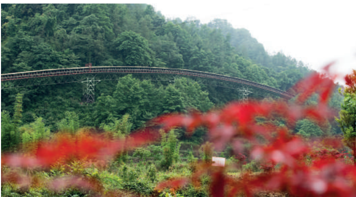
Whenever technically possible, the routing of the conveyor has been adapted to the topography
