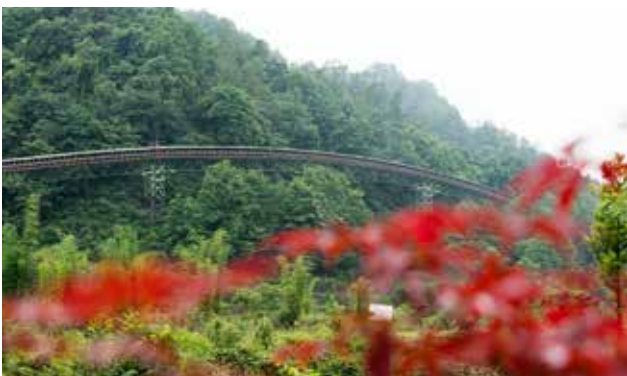
Whenever technically possible, the routing of the conveyor has been adapted to the topography. Photo credits: BEUMER Group GmbH & Co. KG
